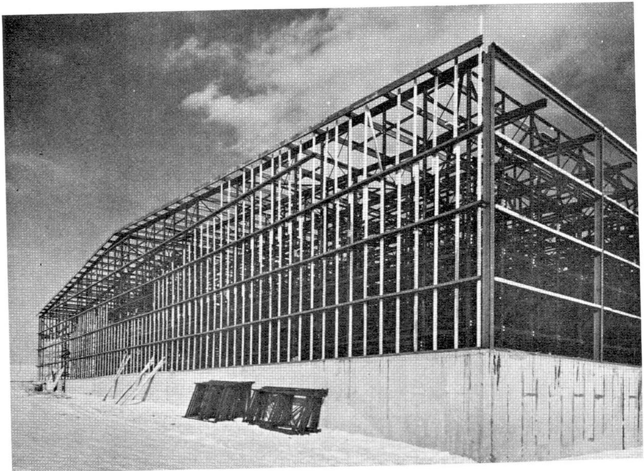
Republic Steel Corporation are producers of complete rack buildings including steel framing and steel panels for sides and roof.
