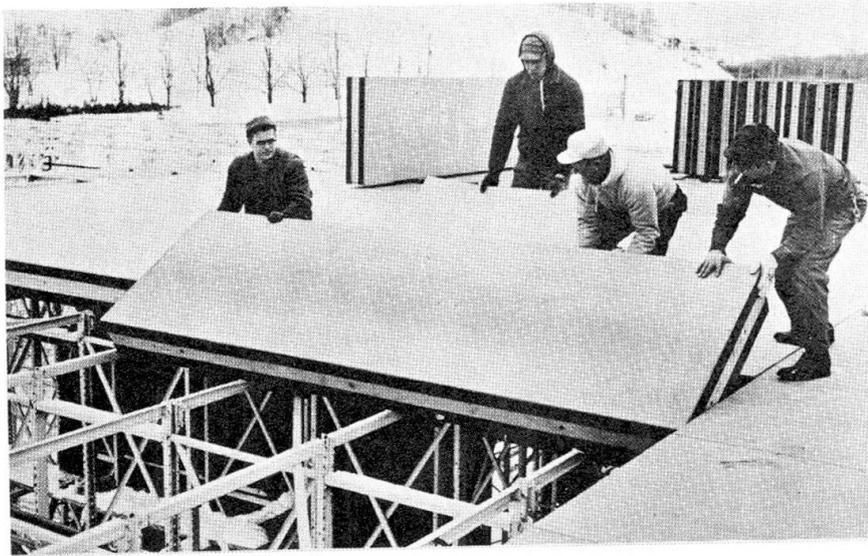
Another example of a rack building is the Potato Service Company building at Presque Isle, Maine. The racks supporting this building are also "drive-in" type. Speed of erection of the total building is another feature of rack buildings.
