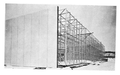
Pre-fabricated wall panels are put in place and bolted together.
