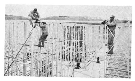
The racks which hold the goods and support the roof, are assembled and lagged to the floor. Here, crew adds bracing over main aisle.
