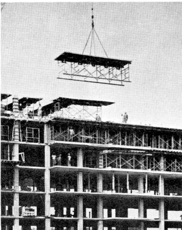
Complete shoring unit is lifted by tower crane to next pour area.
