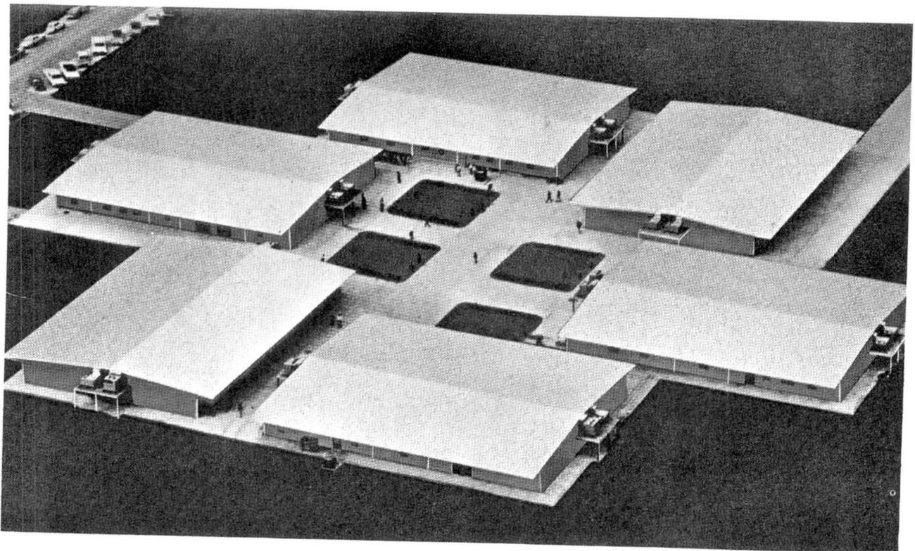
An adaptation of Mobile Homes to schools has been done successfully. Two mobile home units 12' wide by 40' long with one side on each, when assembled side by side provide a very successful classroom 24' by 40'. Steel is used extensively for structural framing and exclusively for underframes. Galvanized sheet steel is used for roofs, heating and ventilating ducts. Steel is also used for some exterior panels.
