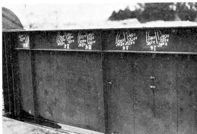
Fig. 11. Location of Cracks Type BM-1 in Girder F-5.
