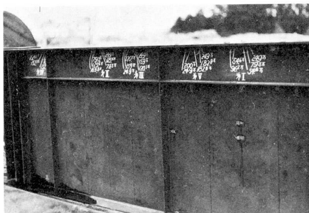
Fig. 11. Location of Cracks Type BM-1 in Girder F-5.
