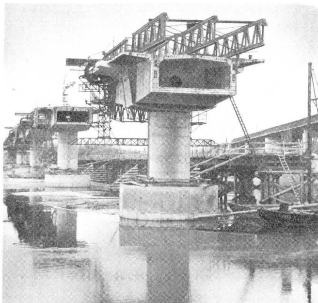
Fig.No.4.:The monolytical concreted cantilever prestressed bridge "KO".
