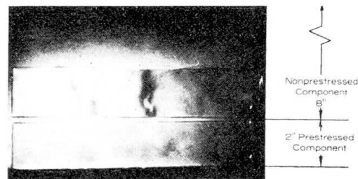
Fig.5. Microcracking in 'S' beam under self load.
