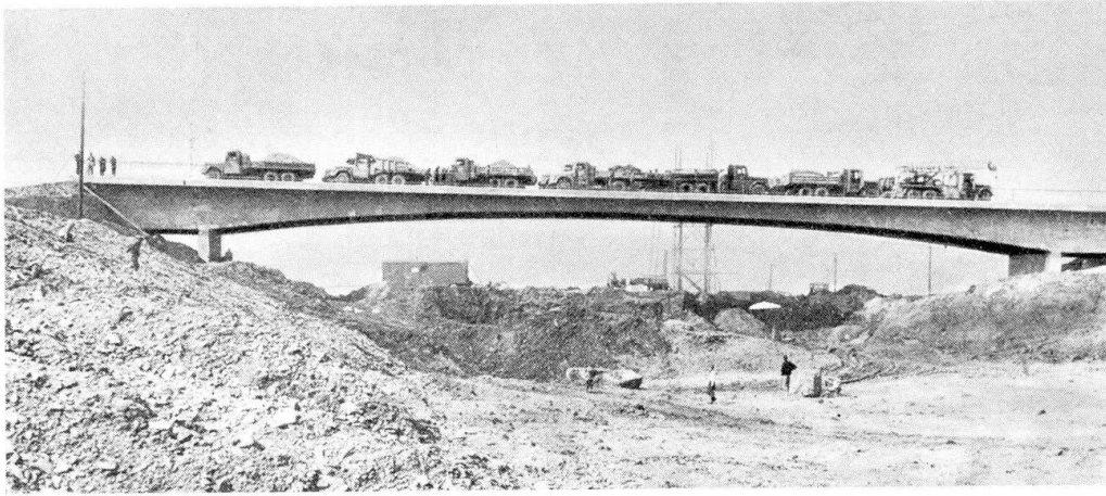
Fig.No.1.:The monolytical concreted framework prestressed concrete highway bridge " K " - Kotešová.
