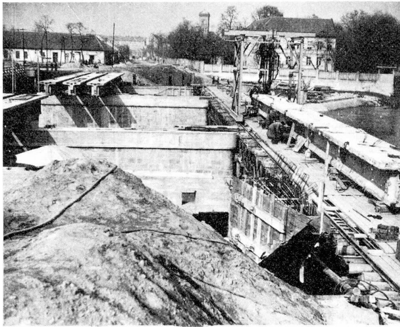
Fig.No.8.:The highway bridge " NZ " with continuous precast prestressed concrete girders during construction.
