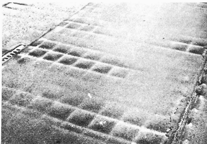
Figure 13: Steel mesh anchoring; plasterlike top surface
