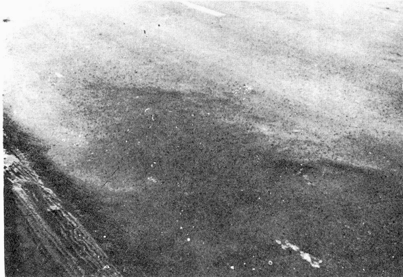
Figure 7: Big-sized shoving, up to 7 cm deep
