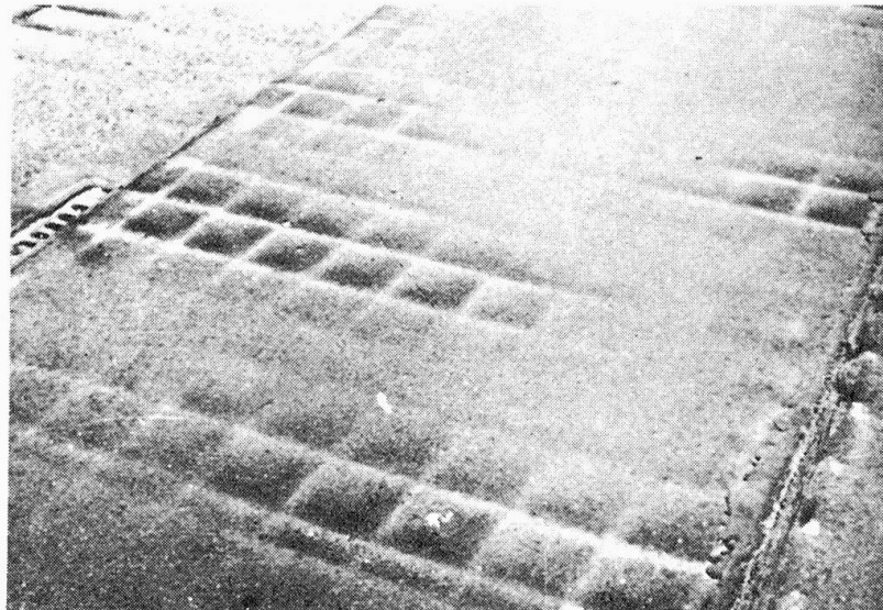
Figure 13: Steel mesh anchoring; plasterlike top surface
