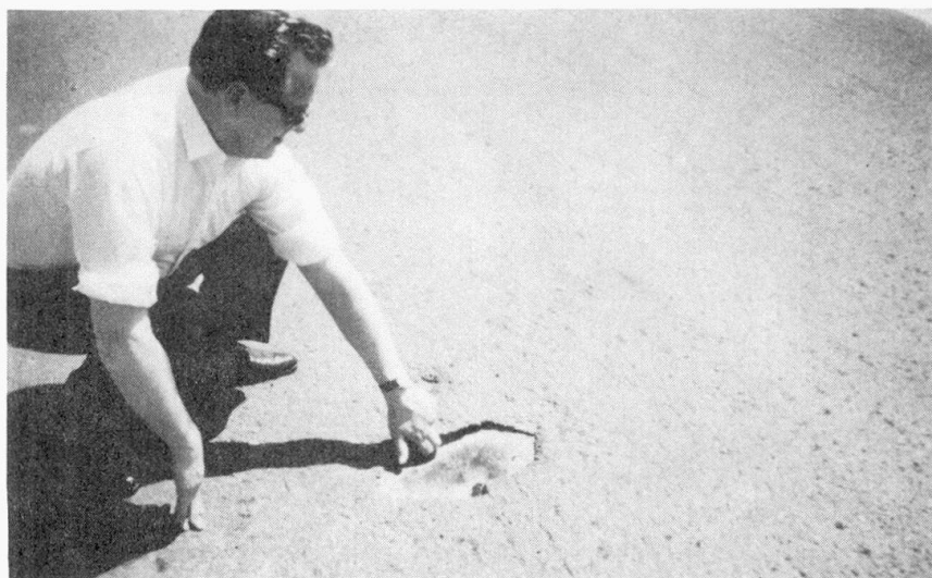
FIGURE 5. BREAKOUT OF WEARING COURSE OVER SPLICE PLATE ON CONCORDIA BRIDGE AFTER TWO YEARS OF SERVICE
