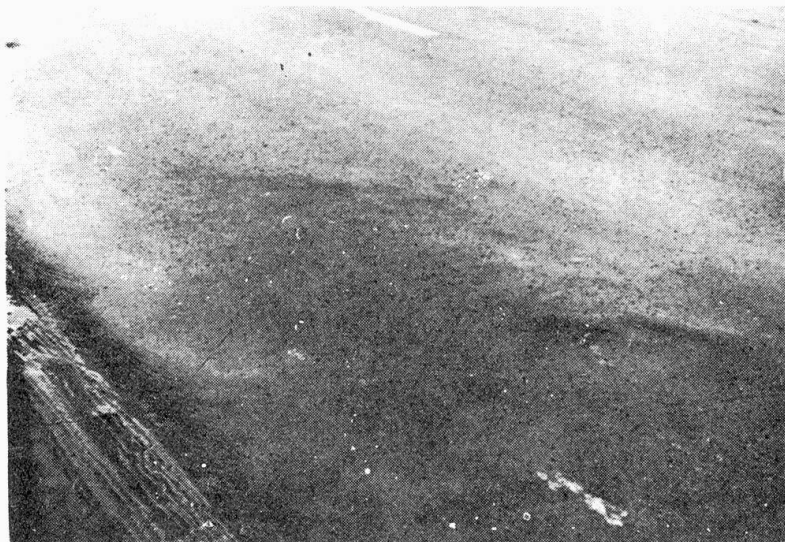
Figure 7: Big-sized shoving, up to 7 cm deep
