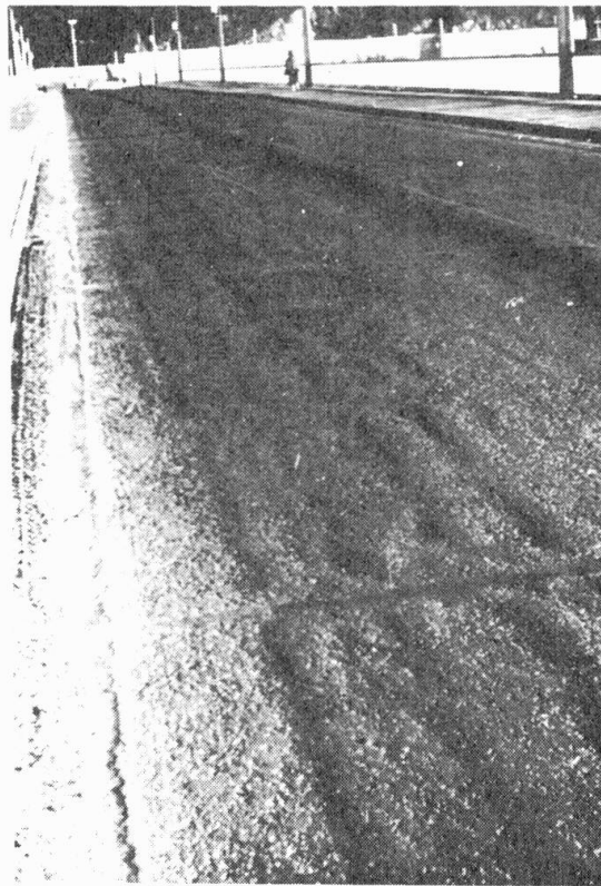
Figure 6: Rutting (transverse waving)
