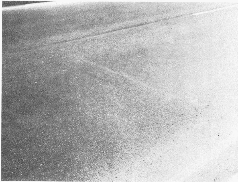
FIGURE 1. SLIGHT UNEVENNESS IN THE SURFACE COURSE OVER THE SPLICE PLATES ON THE PORT MANN BRIDGE AFTER 2-1/2 YEARS IN SERVICE
