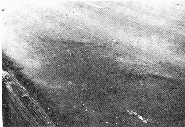
Figure 7: Big-sized shoving, up to 7 cm deep
