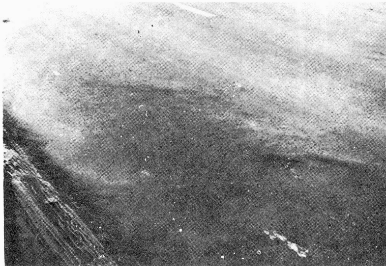
Figure 7: Big-sized shoving, up to 7 cm deep
