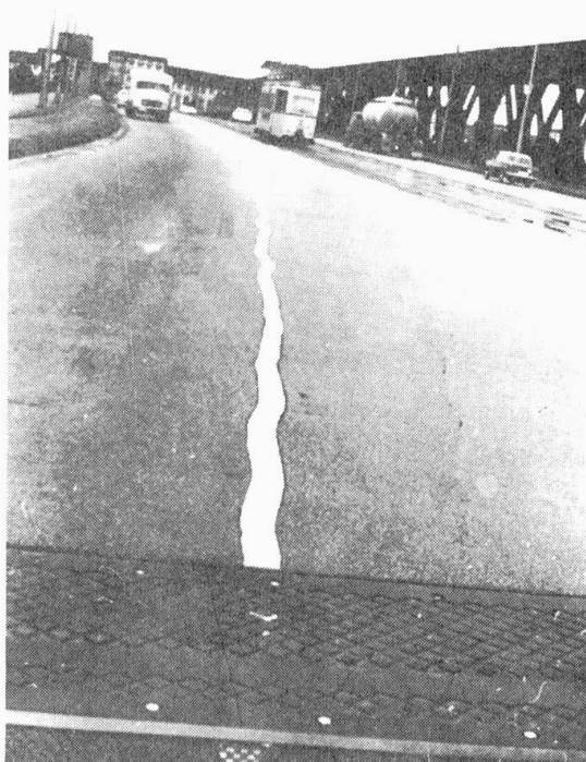
Figure 10: Shoving visible from deformed marking strip
