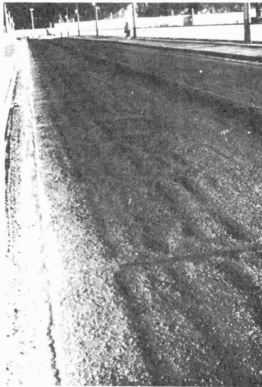
Figure 6: Rutting (transverse waving)
