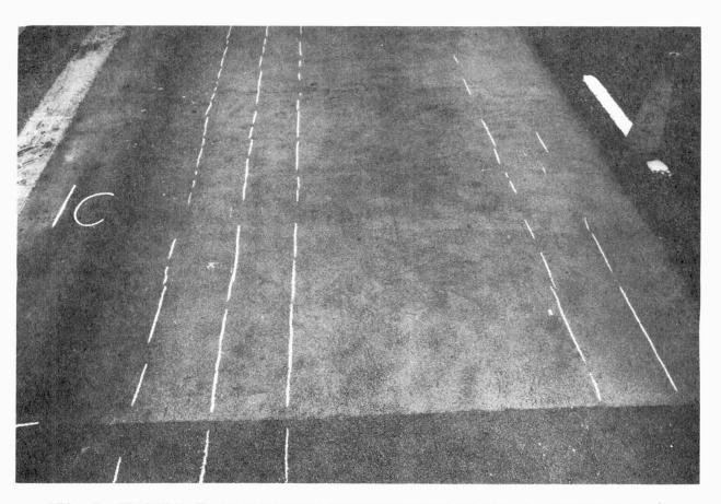
FIG. 5 CRACKING IN EPOXY RESIN SURFACING ON SECTION 1C, NOVEMBER, 1967
