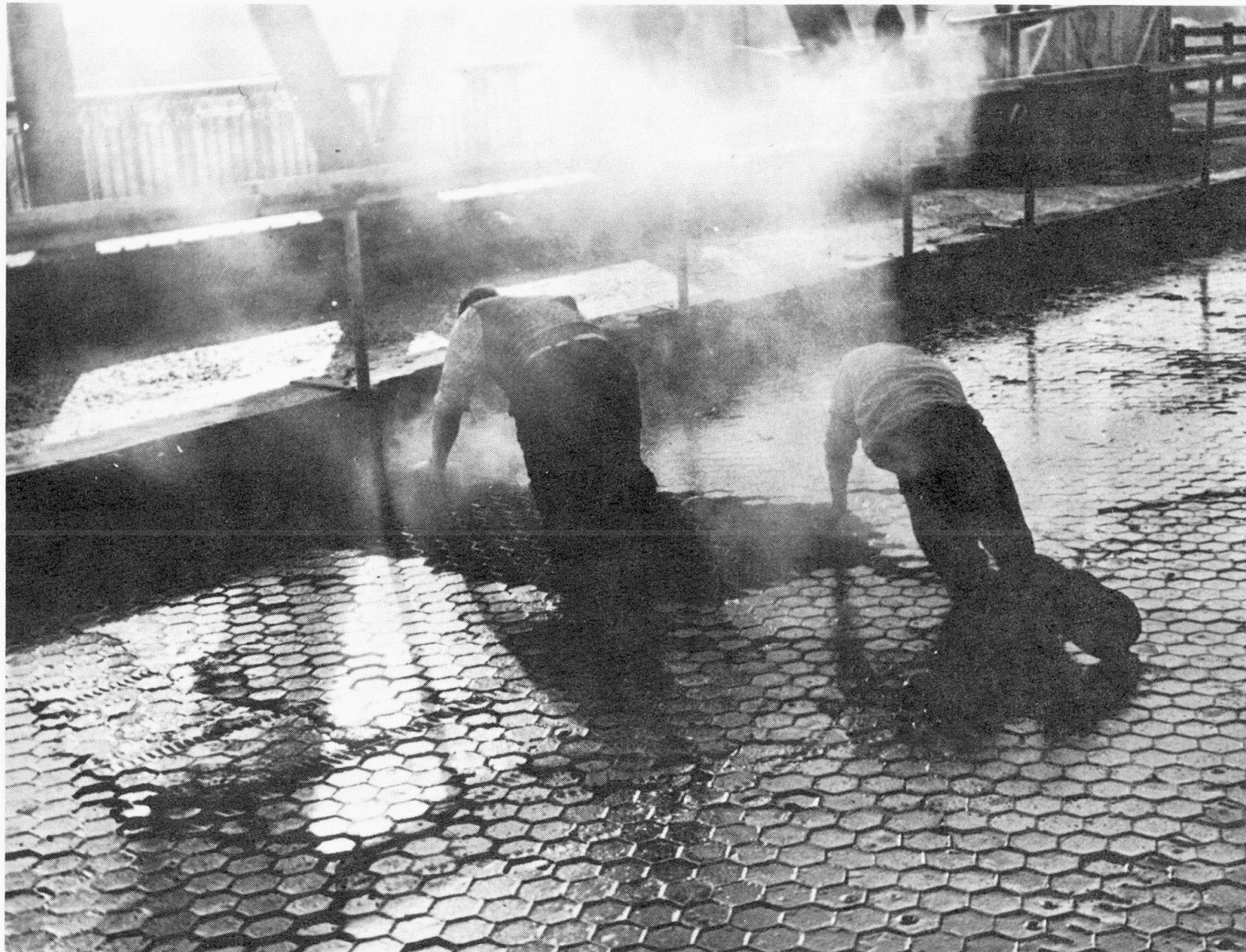
FIG. 1 HEXAGONAL GRID 1 in (25 mm) DEEP, ON AN ALUMINIUM DECK OF A BASCULE BRIDGE IN HULL.
