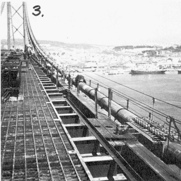
Photograph 3 shows some additional details of the grid floor which will be filled with concrete.
