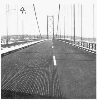
Photograph 4 shows the completed bridge deck of the Tagus River Bridge. The left lane has an open grid floor and the right lane has a concrete filled grid floor.
