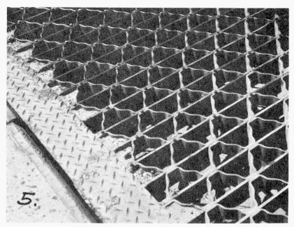
Photograph 5 shows an open grid on a bascule bridge in Connecticut which has a hexagonal pattern. This photograph also shows the modification which has been made to improve traction. One quarter inch round studs have been welded on the top of the longitudinal bars to give a rough texture. A portion of the floor on the lower right does not have the additional studs.
