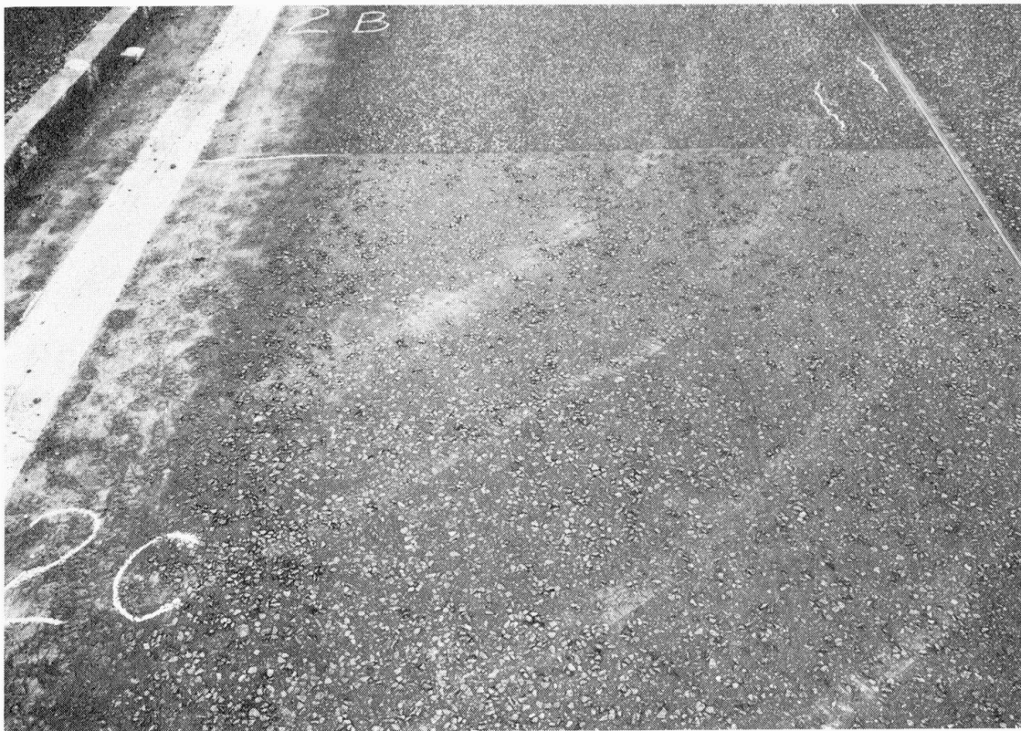
FIG. 7 MASTIC ASPHALT ON FILLED RUBBER BITUMEN, NOVEMBER, 1967
