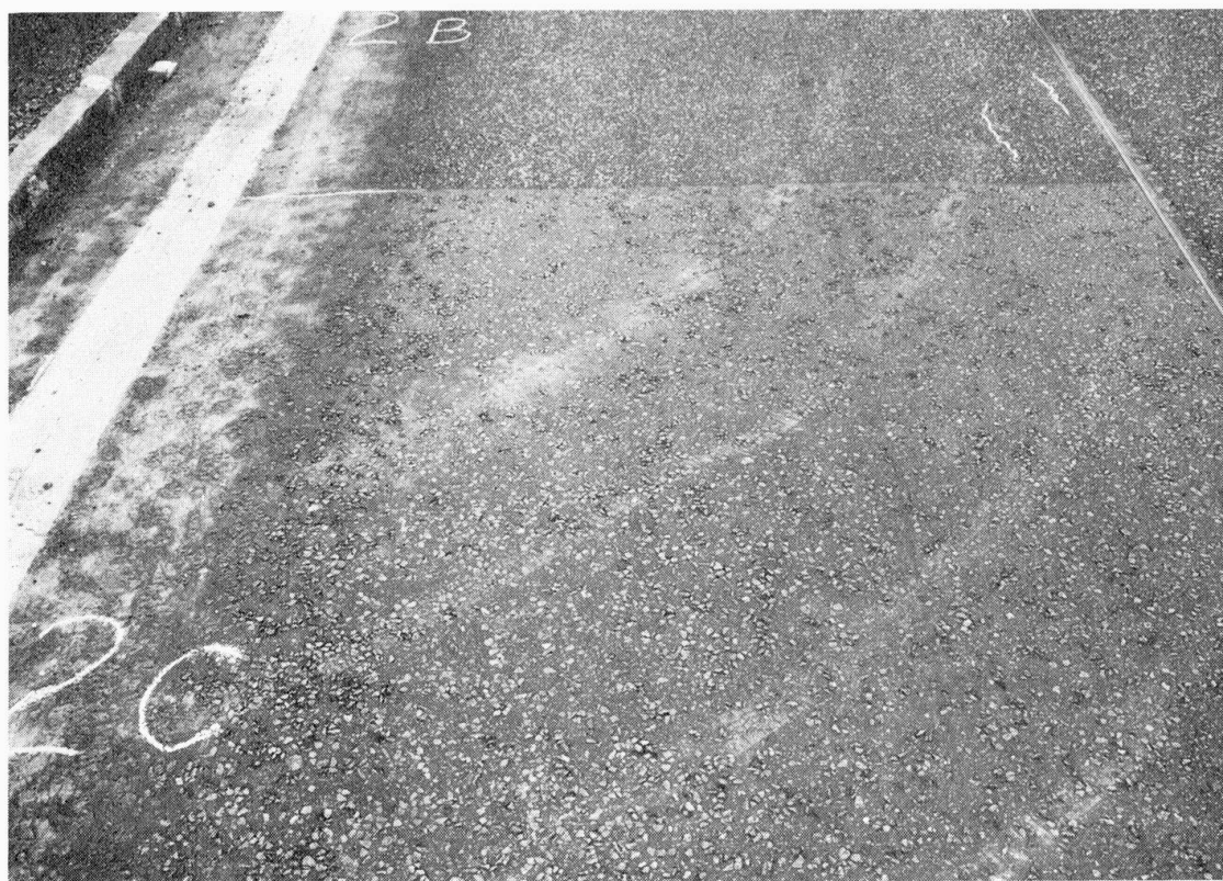
FIG. 7 MASTIC ASPHALT ON FILLED RUBBER BITUMEN, NOVEMBER, 1967
