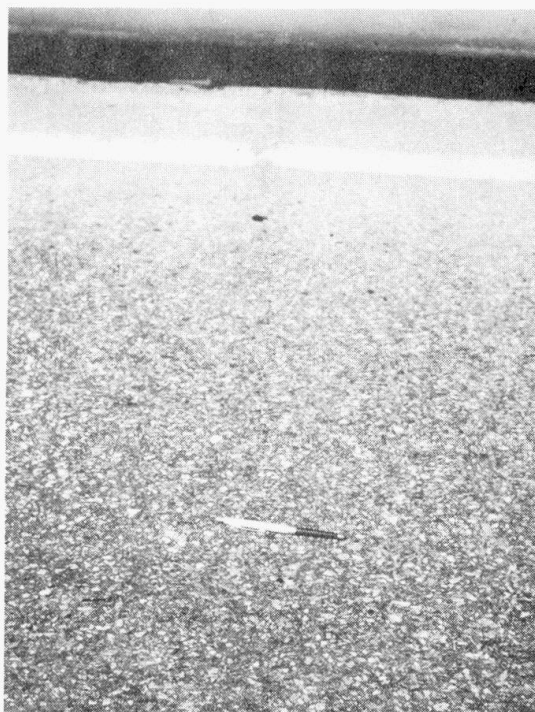
FIGURE 1. SLIGHT UNEVENNESS IN THE SURFACE COURSE OVER THE SPLICE PLATES ON THE PORT MANN BRIDGE AFTER 2-1/2 YEARS IN SERVICE
