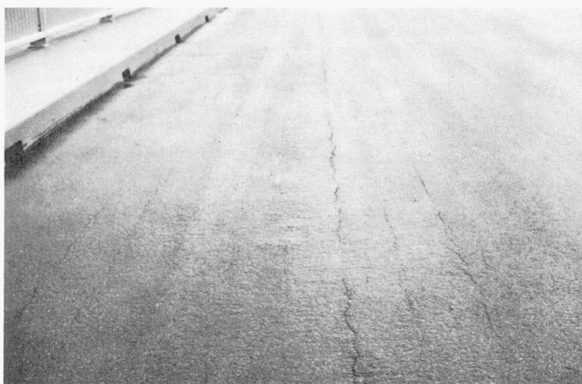
FIGURE 4. LONGITUDINAL CRACKS IN THE ACPAVEMENT ON THE CONCORDIA BRIDGE AFTER TWO YEARS IN SERVICE
