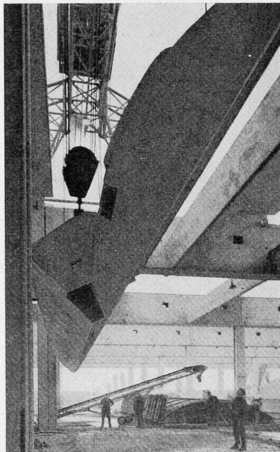
Fig. 3 - Alfa-Romeo factory, Arese (Impresa ICIS). Placement of a precast thin shell.
