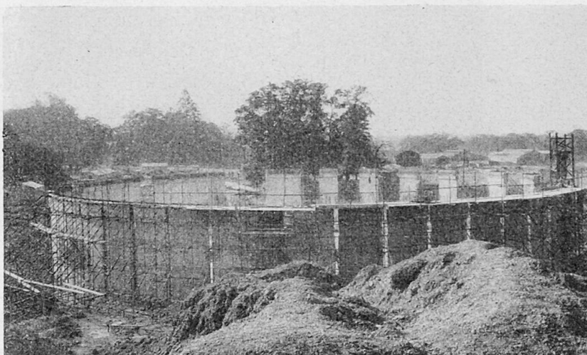
Fig. 12 - 160 ft dia. tank at Windsor using precast units cast on site.
