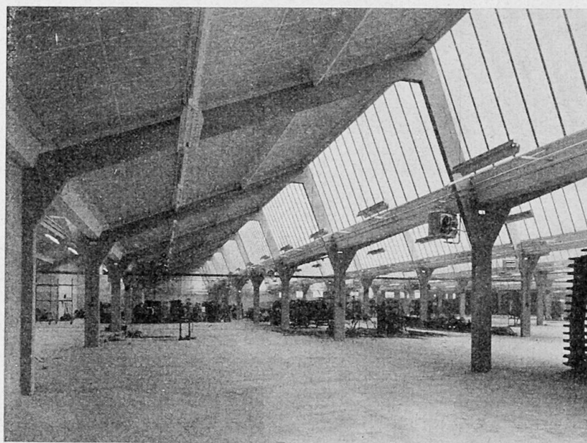
Fig. 5 - Precast northlight framework for factory at Bracknell New Town.
