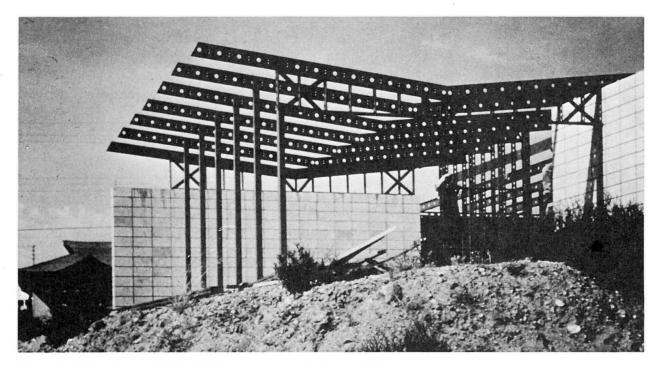
Fig. 6 Cold-Formed Steel Framing: Joists and Studs
