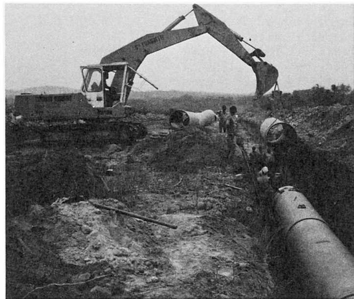
Fig.15 Laying of FRP-pressure pipeline in Africa (Constr.by Durit-Werke, Kärnten, Austria)
