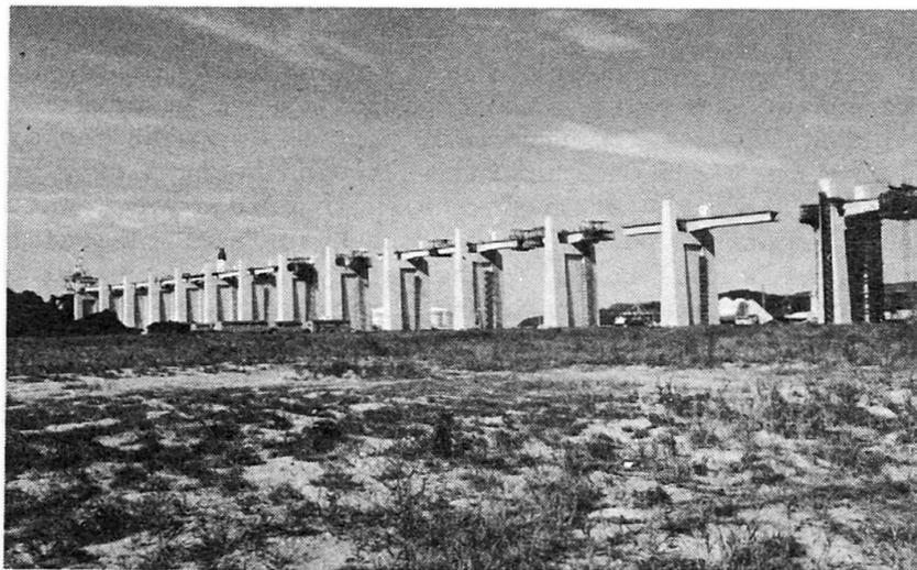
Fig. 18 Construction of Bannosu Viaduct
