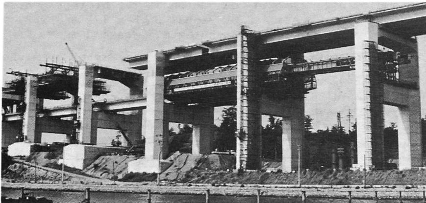
Fig. 11 Erection by Movable Staging for Lower Girder
