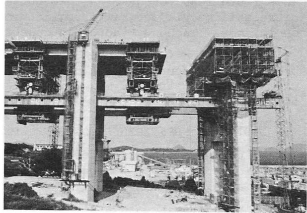
Fig. 3 Erection by Movable Staging
