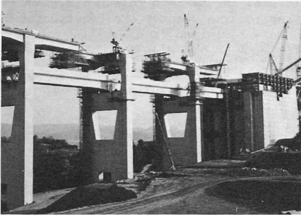
Fig. 2 Cantilever Erection
