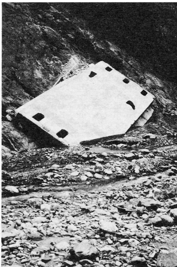
FIG. 2 200 Ton Bridge slab after the flash flood.
