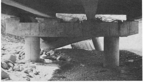
FIG. 7 Support structure damaged by the flash flood.
