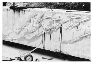
Fig. 18 Example of Crack Grouting
