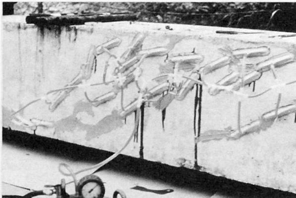
Fig. 18 Example of Crack Grouting
