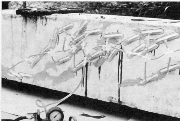
Fig. 18 Example of Crack Grouting
