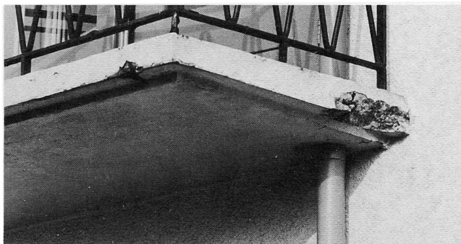
Fig. 6 Corrosion damage due to carbonation
