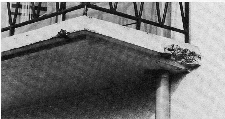
Fig. 6 Corrosion damage due to carbonation
