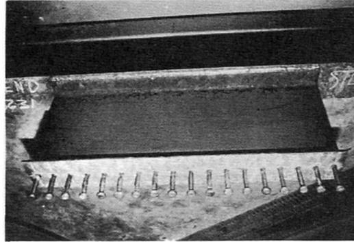
Fig.2 Headed stud arrangement used for phase one
