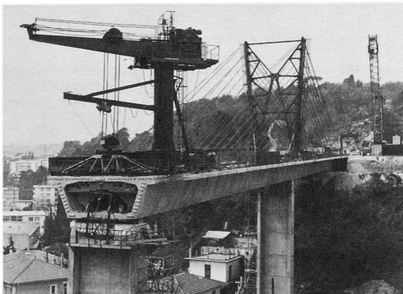
Fig. 3 - The mast and the stay arrangement
