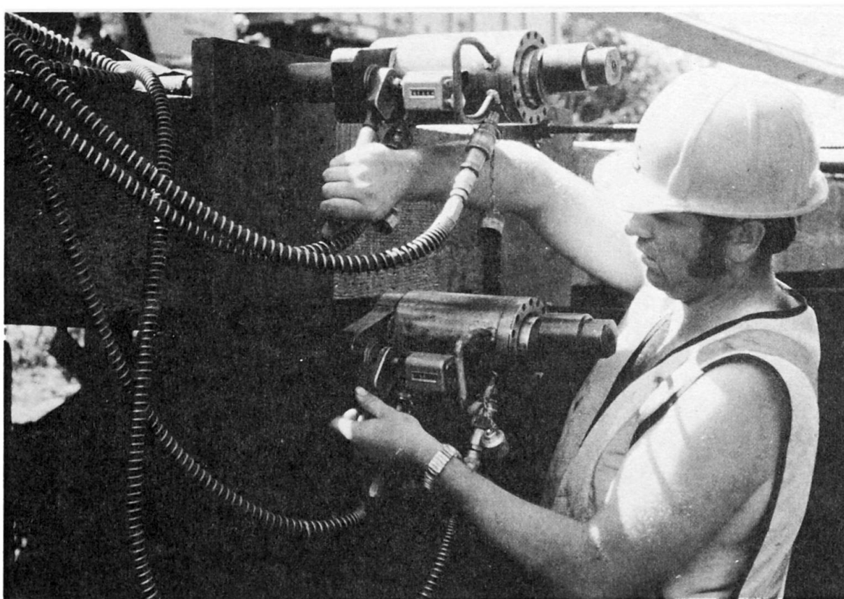
Figure 6 Prestressing of Hebert Creek Bridge
