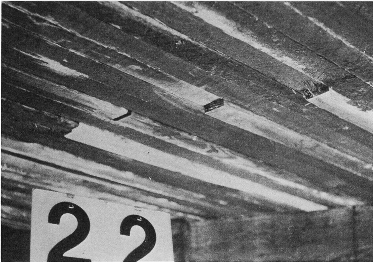
Figure 12 "Piano-Key" Failure of Nailed Decks with Butt-Joints
