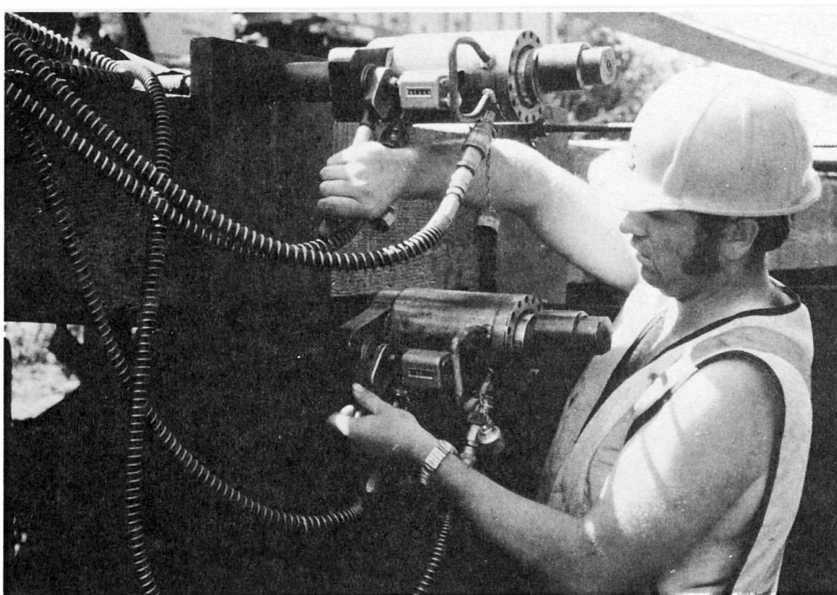
Figure 6 Prestressing of Hebert Creek Bridge
