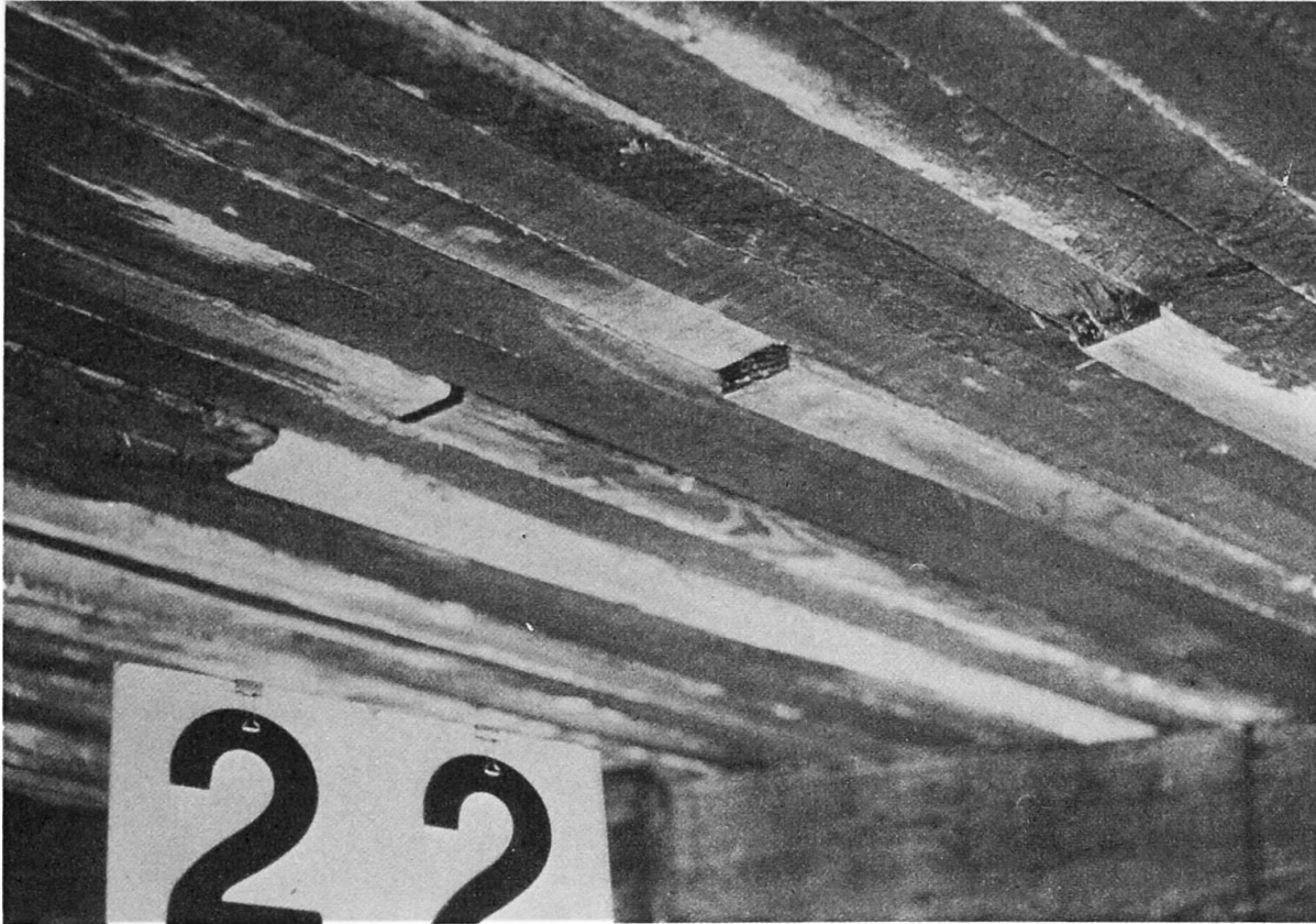
Figure 12 "Piano-Key" Failure of Nailed Decks with Butt-Joints
