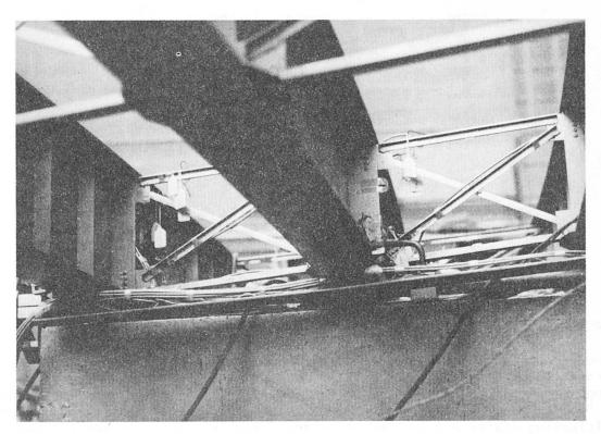
Fig. 14 Intermediate Diaphragm at Center Pier
