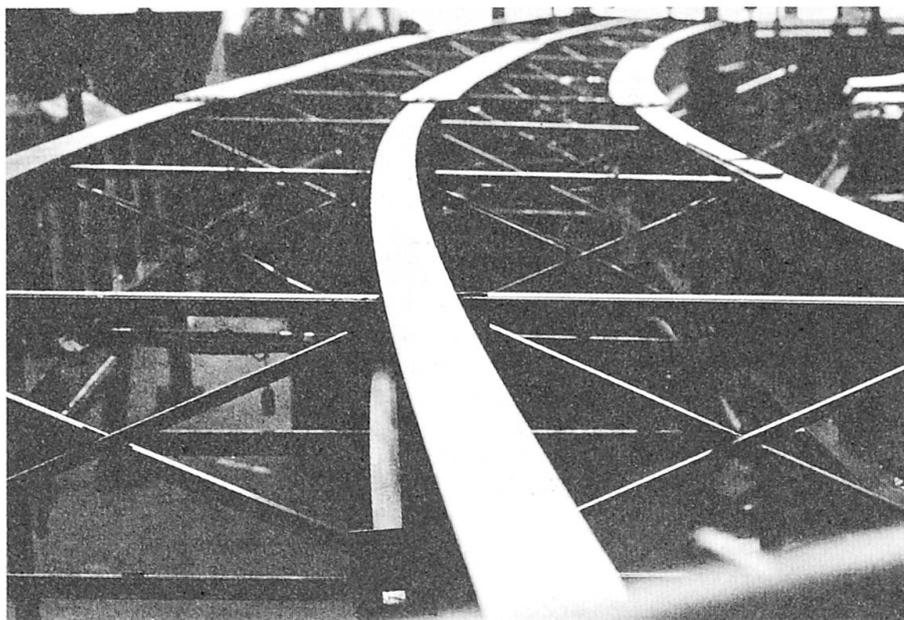
Fig. 8 Intermediate Diaphragms
