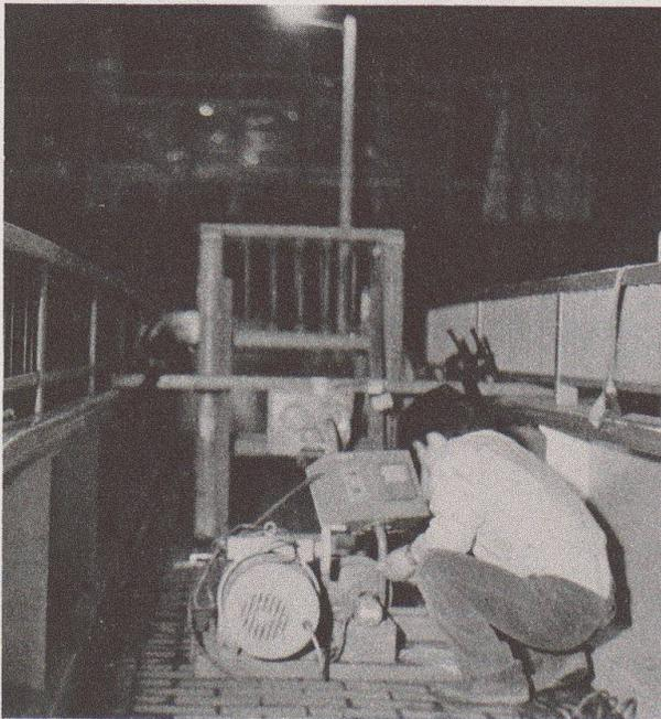
Picture 1 Experimental absorber installed on Shibuya-1-chome footbridge
