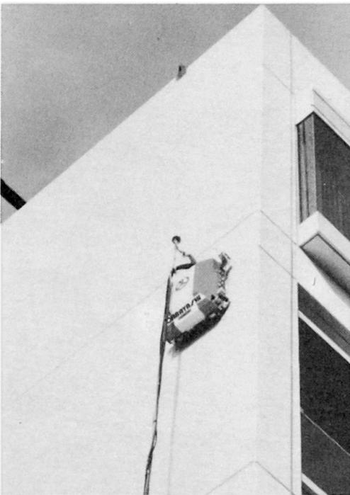
Photo 21 Wall inspection robot
