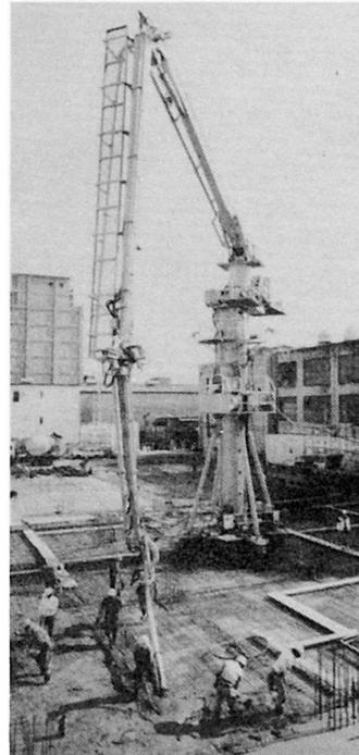
Photo 5 Placing crane
