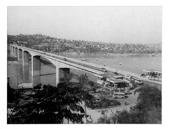
near the pier for main span is ll m in height. The thickness of its walls is 27 - 40cm. During construction the water level was 165m, with 2.5 m/sec. of flow velocity. For construction of the bridge, 117'000 m3 of earth and stone was excavated and 81'600 m3 of concrete cast.
