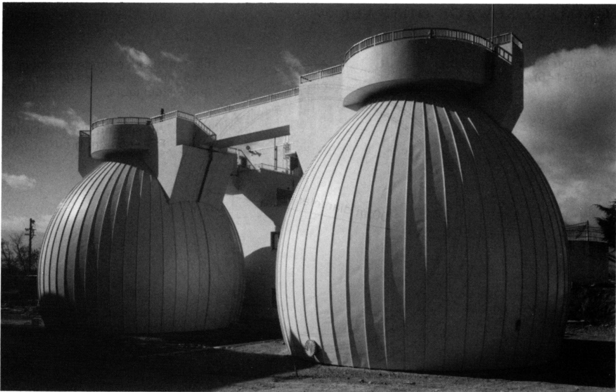
Fig. 6 View of the completed tanks
