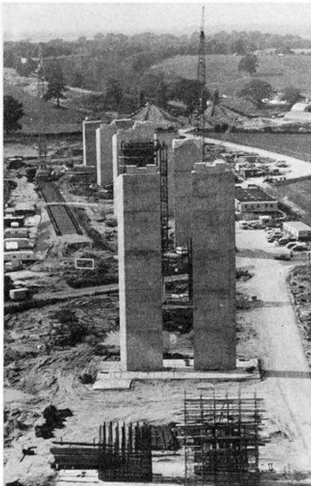
Viaduct piers – August 1980
