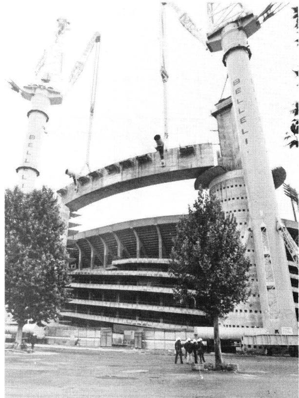
Fig. 6: Lifting a main box girder
