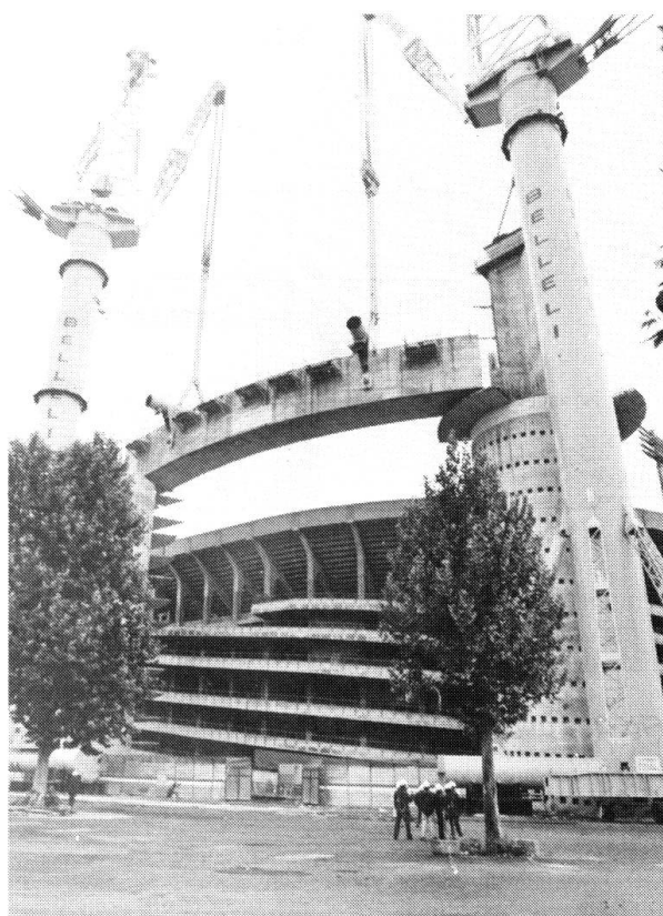
Fig. 6: Lifting a main box girder
