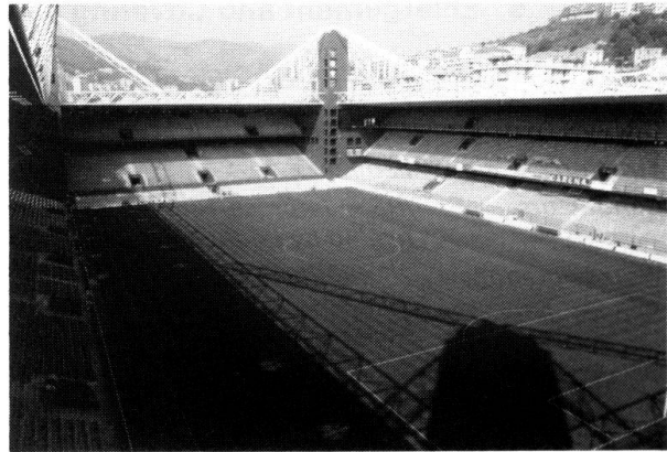
Fig. 3: Inside view of the Stadium
