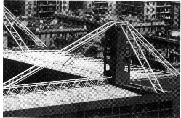
Fig. 2: Detail of corner building
