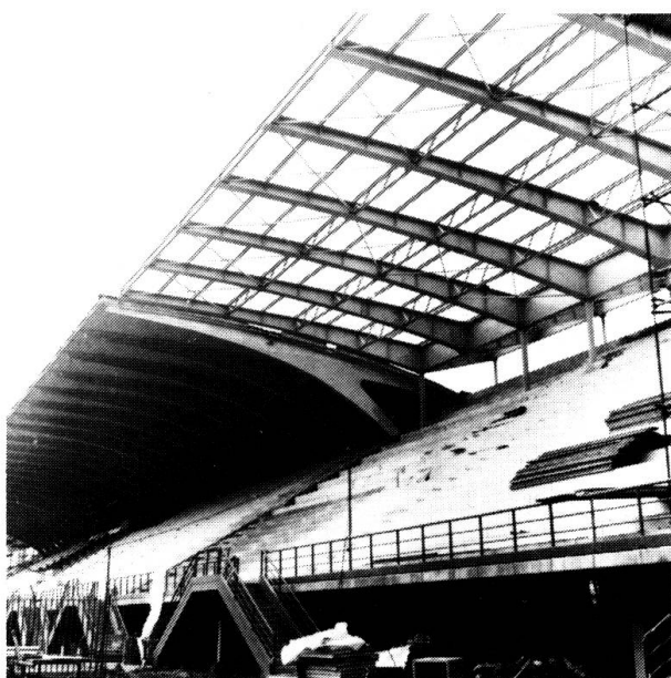
Fig. 1: New cantilever steel cover
