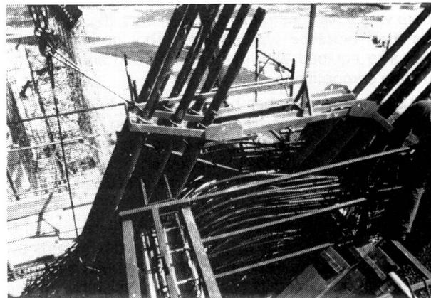
Fig. 4: Cantilevers' connection joint during construction (partial view)
