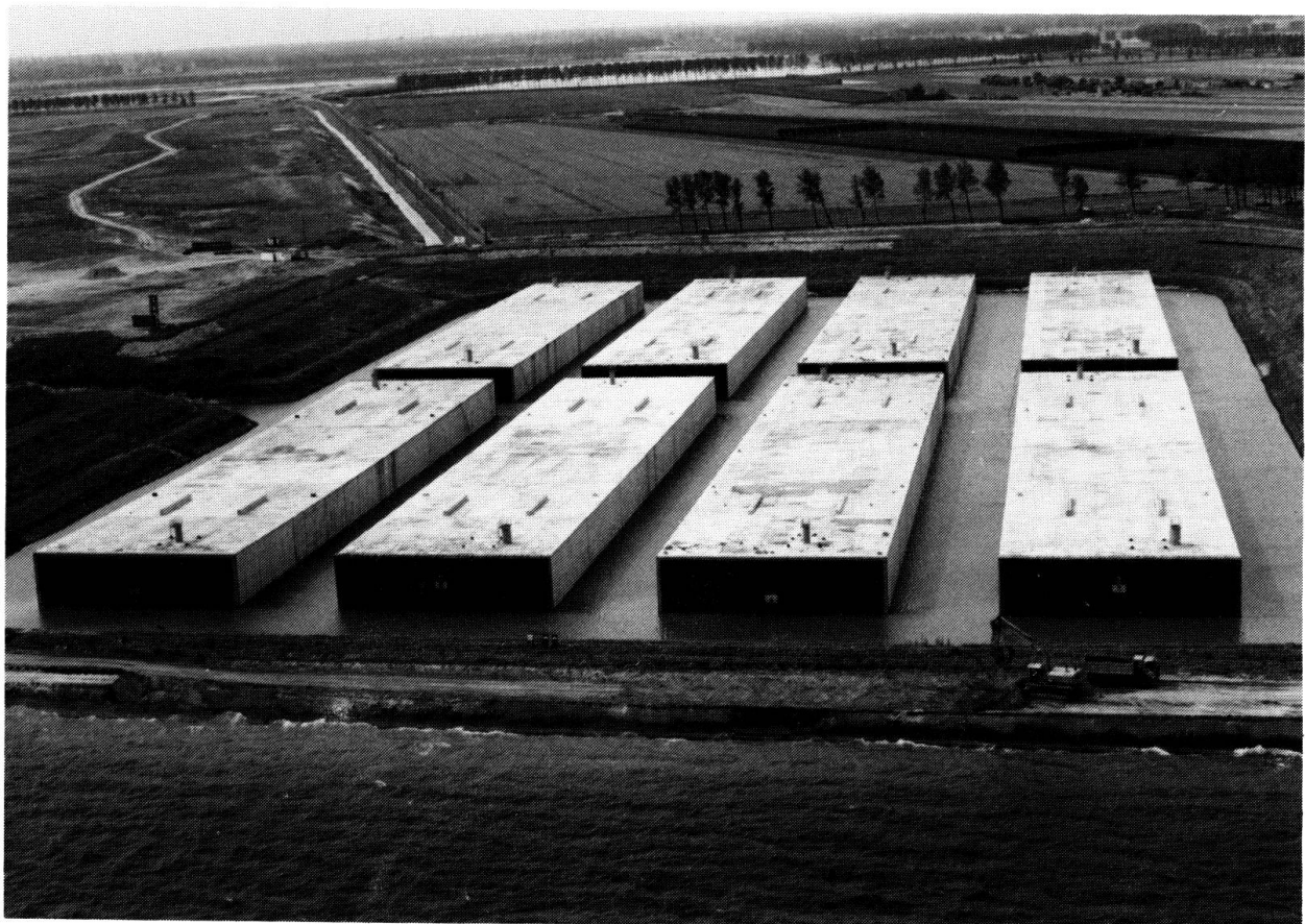
Fig. 1: View of the construction dock
