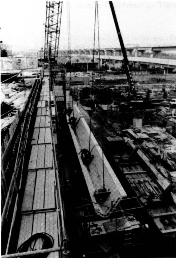
Fig. 3 Assembly of post-tensioned panel on site
