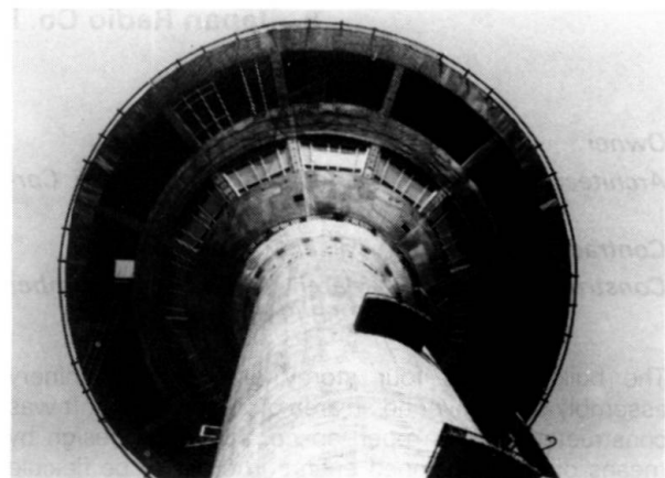
Fig. 3 Bottom view of skypod floor
