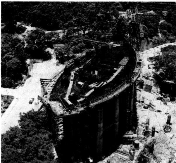
Fig. 4 Transfer plate of Tower B under construction (June 1988)
