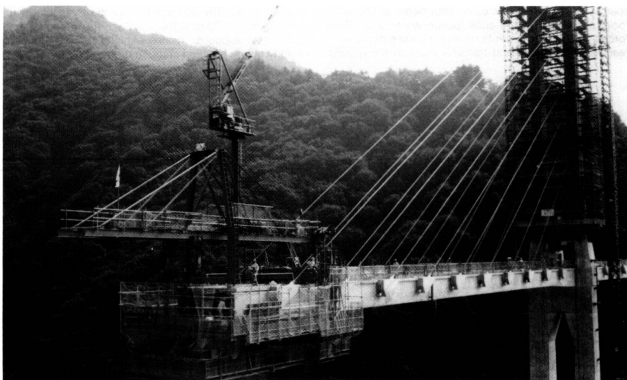
Fig. 4 View of the Suspended Long Traveller (SLT)
