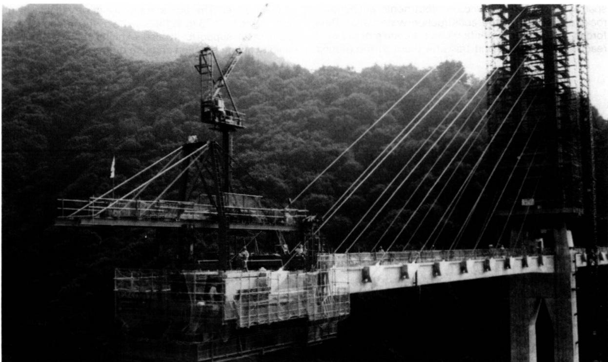
*Fig. 4 View of the Suspended Long Traveller (SLT)*
