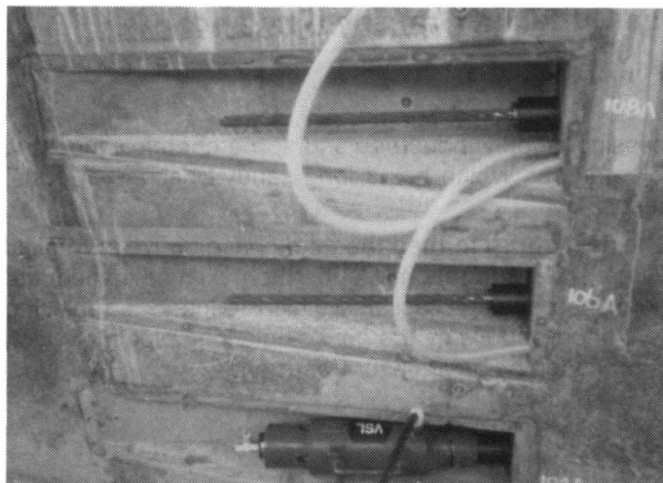
Fig. 5 Anchorages and stressing of horizontal shell tendons
