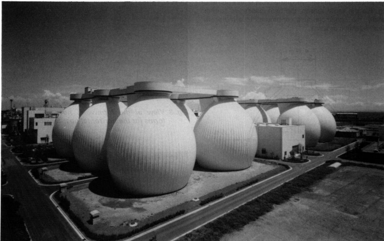
*Fig. 4 Prestressed concrete digester tanks*
