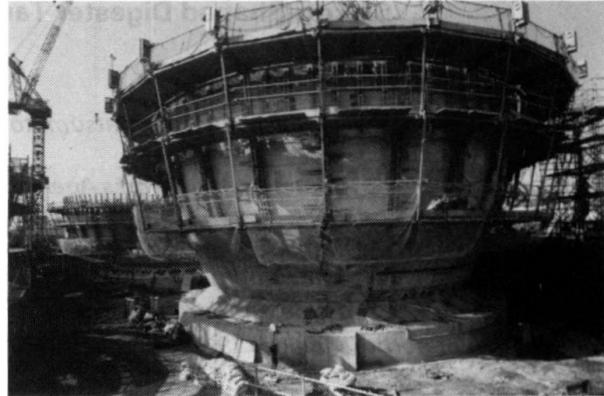
*Fig. 3 Construction by jump form method*
