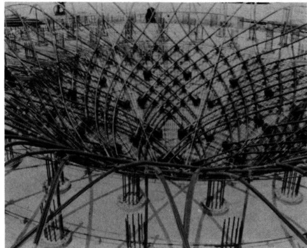
Fig. 2 Helically positioned tendons
