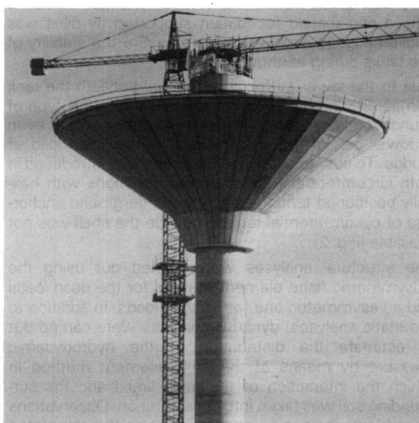
Fig. 6 View of the watertower Caronno after lifting of the bowl
