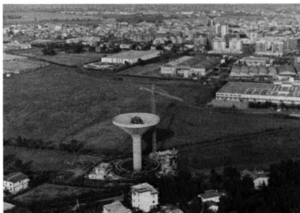
Fig. 1 The watertower at Aprilia during lifting of the bowl
