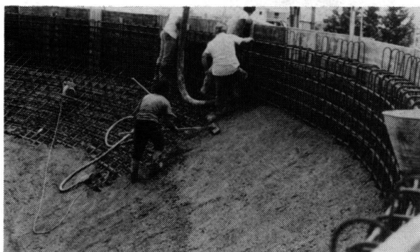
Fig. 4 Concreting of the ordinarily reinforced bowl of the watertower Cisterna
