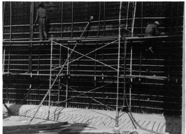
**Fig. 3** Placing of cable ducts in a wall segment
