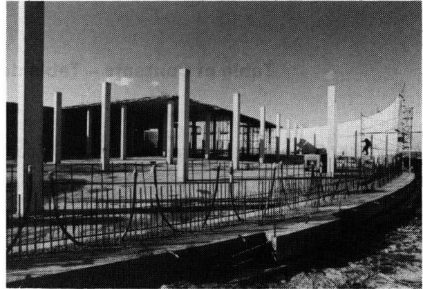
**Fig. 2** View of one of the tanks under construction; in the foreground VSL loop anchorages type L for the vertical wall tendons and a buttress with cables of the ring foundation can be seen
