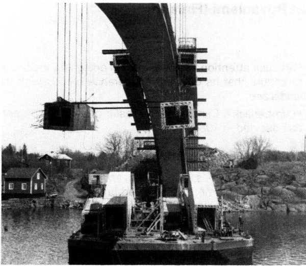
Fig. 4 Erection of the arch elements
