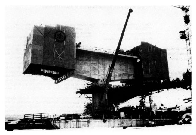
Fig. 2 Cantilever formworks with heat insulation
