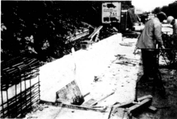
Fig. 3 Working on reinforcements for the construction of the new parapet
