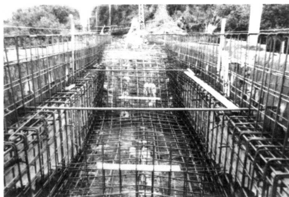
Fig. 3 Arrangement of steel-bars
