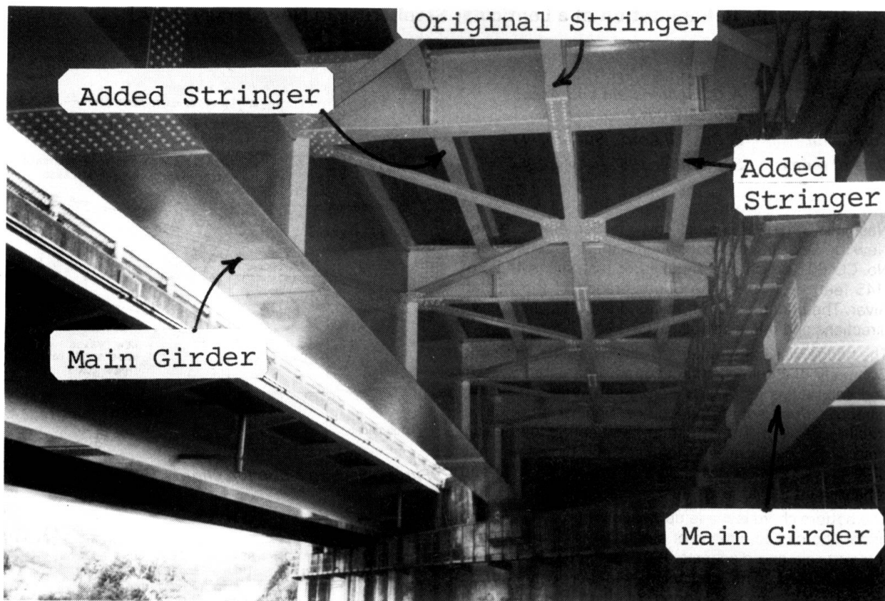
Photo 1 General View of Strengthening
