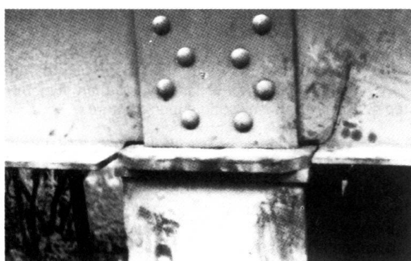
Fig. 5 Crack at stiffening girder web
